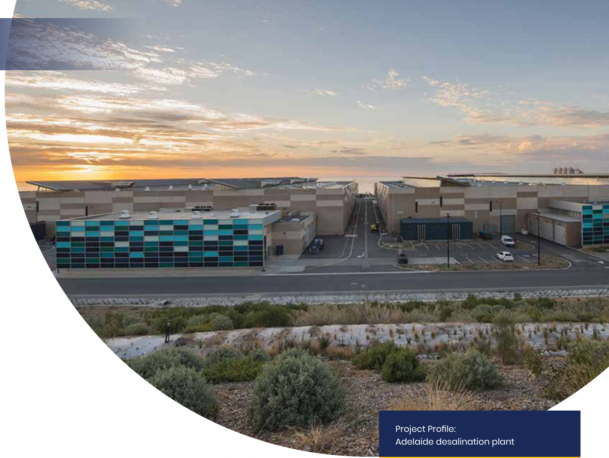
Adelaide desalination plant. Hurricane HI
