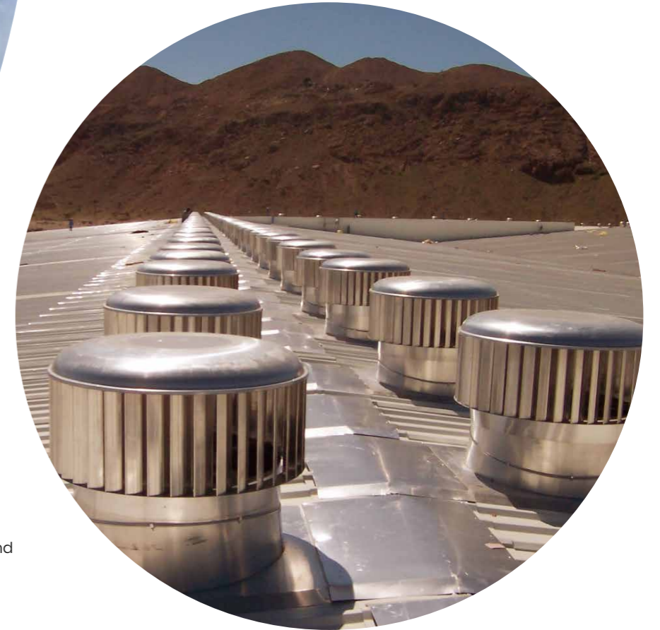
Toyota Spare Parts facility in Muscat Oman, Hurricane H900 for high ambient conditions >40°C.
