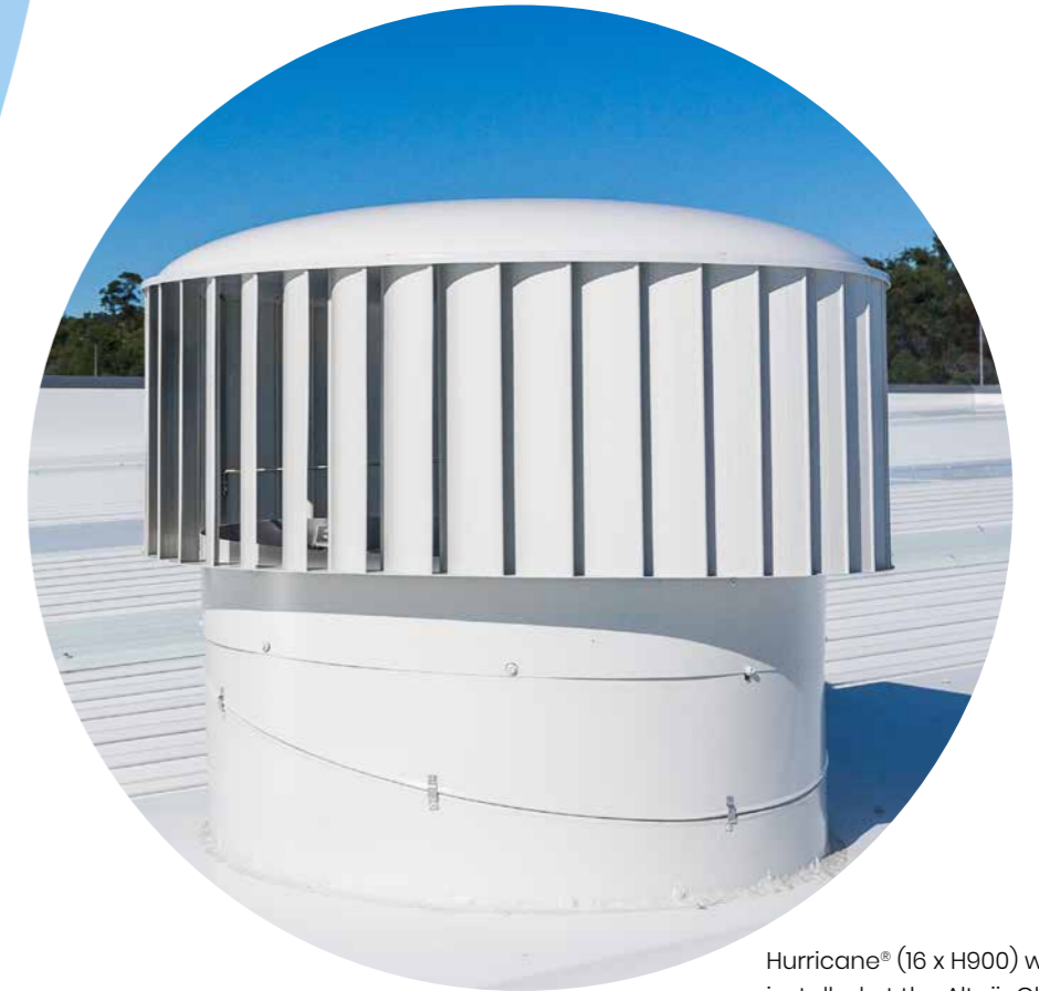
Hurricane® (24 x H800) was installed at the Brisbane Markets to reduce the level of moisture in the air.
