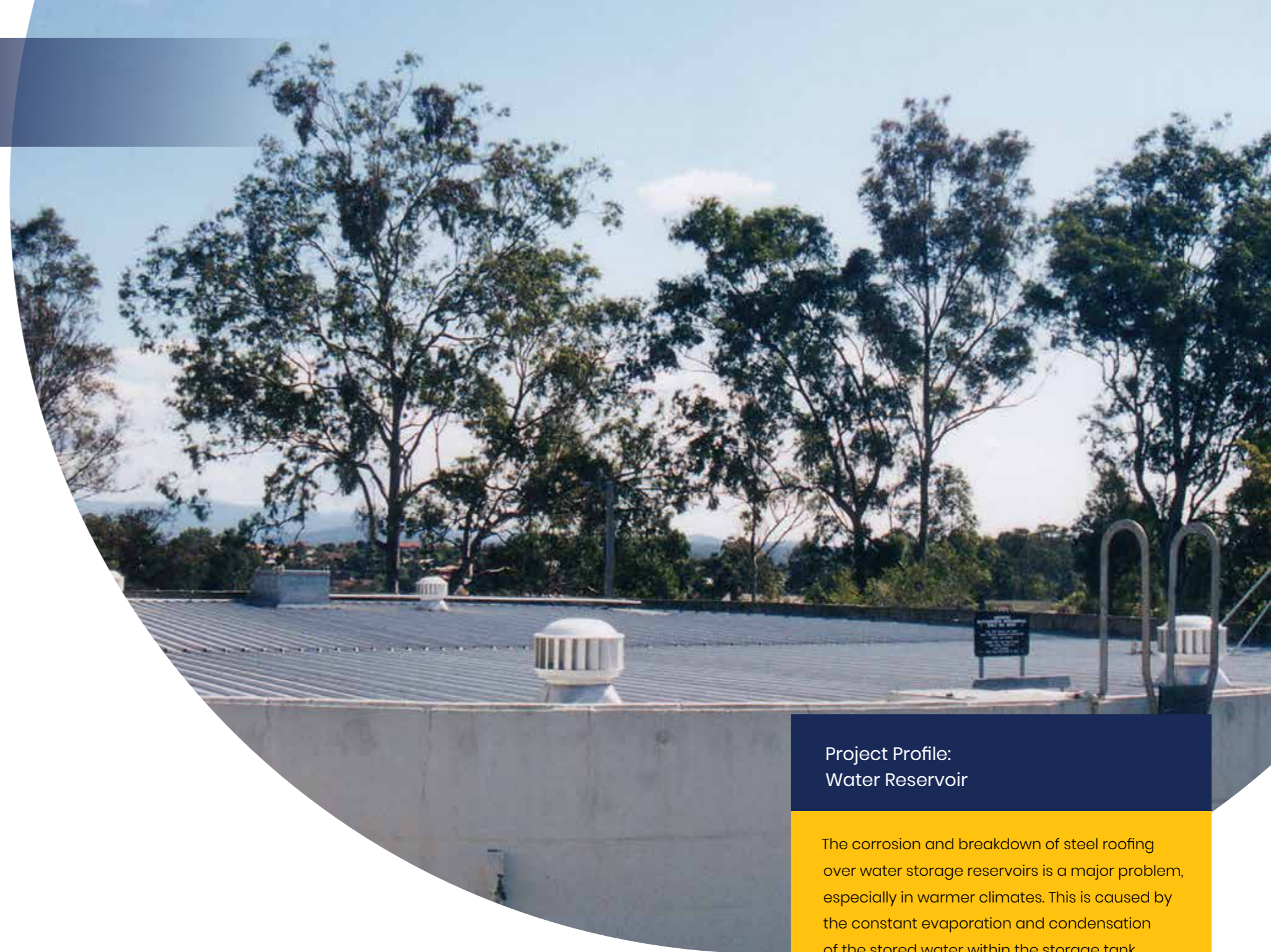
Water Reservoir Installation. Hurricane S2
